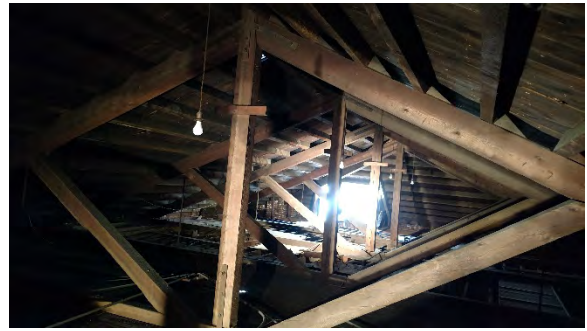
Photo S-1: Existing roof trusses visible in the attic.
